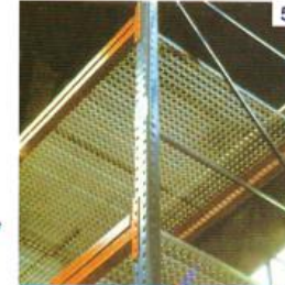
5 Shelf grating with notched T-shaped banding at the Porsche High Rack Warehouse In American university
